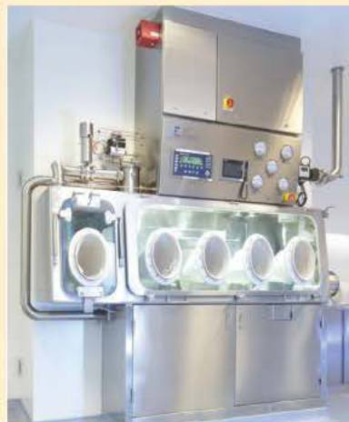
Figure 4 Isolator installed for ADC payload handling
