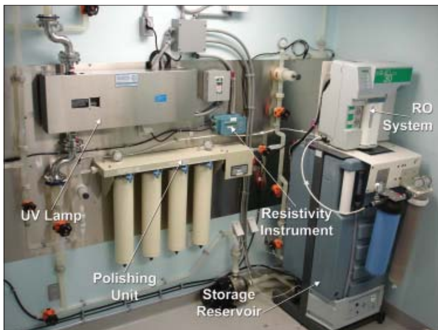
Figure 2. Purified water system: major components.
