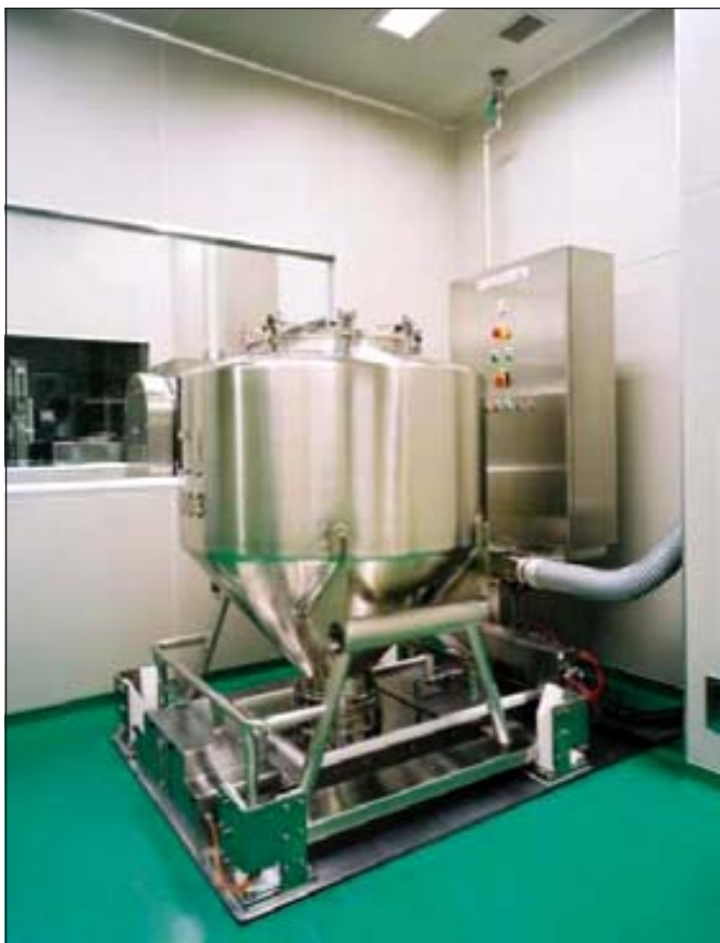
Figure 2. Outside view of docking station.
